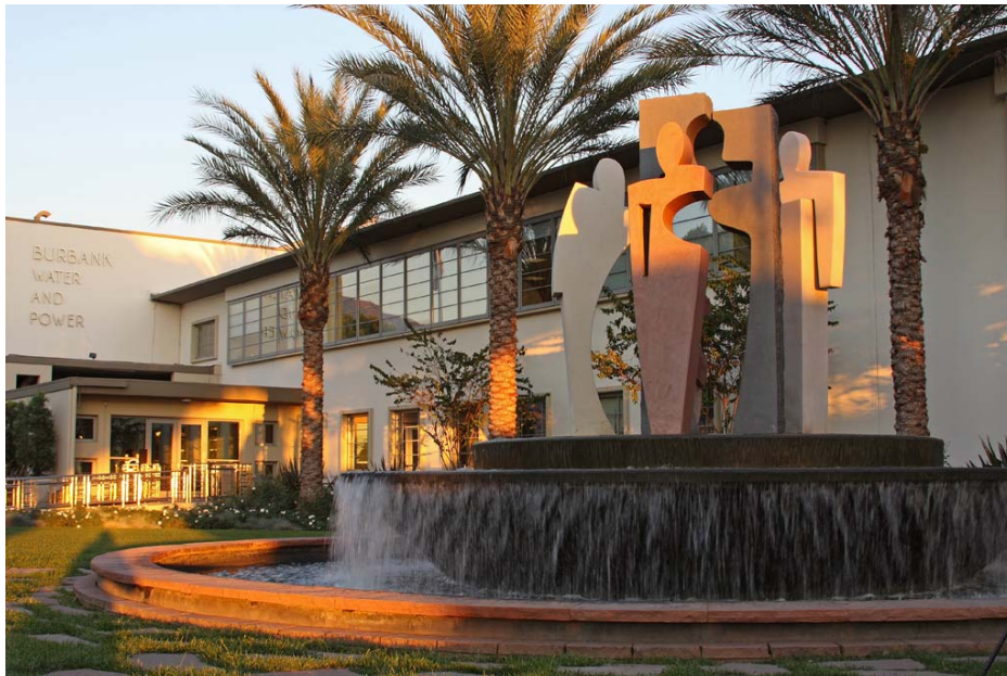
"COMMUNITY FOUNTAIN", BURBANK WATER & POWER, BURBANK, CALIFORNIA
